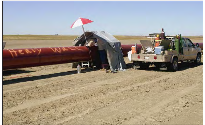
Cross-country pipe welding.
